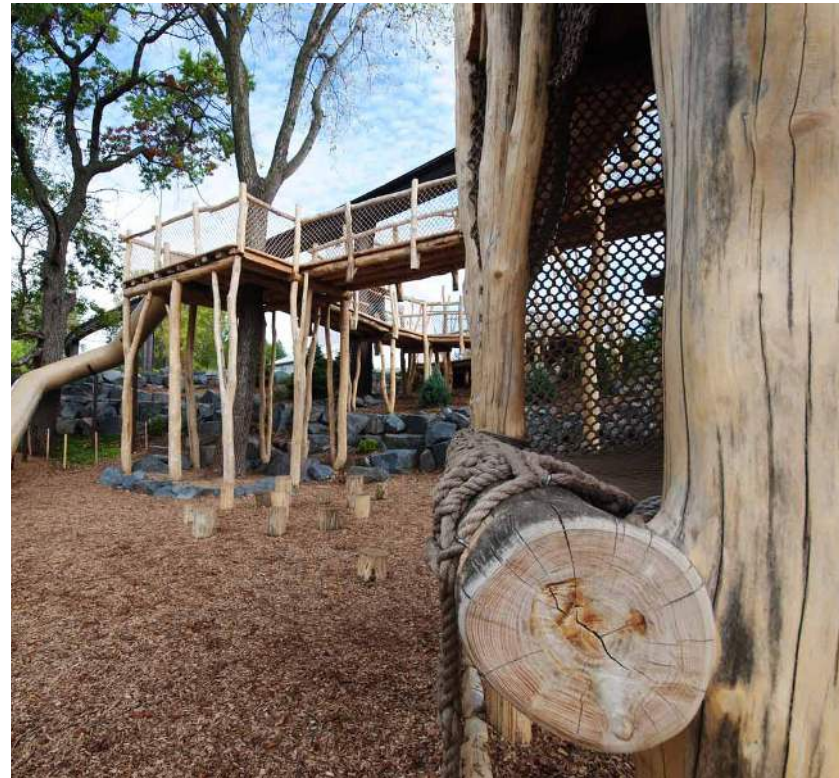
Figure 1. A Black locust tree walk with a hemp-oil based finish, two months after initial application.
