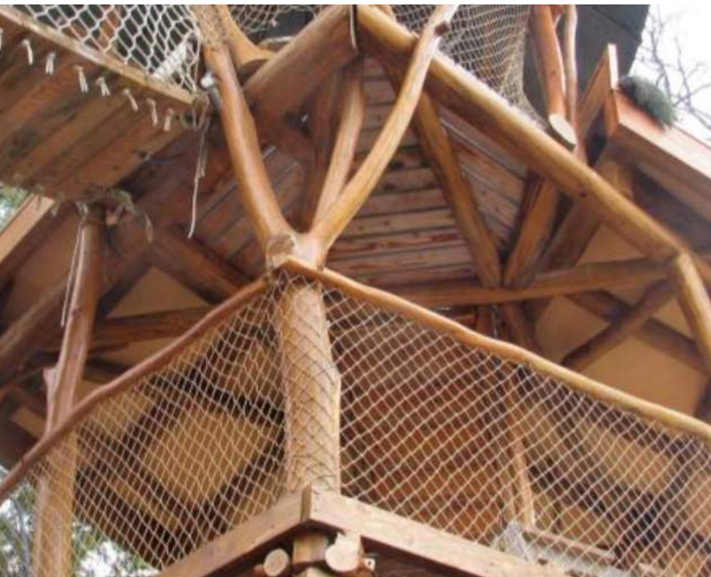
Figure 2. Black locust with a tinted finish, approx. two years after initial application.
