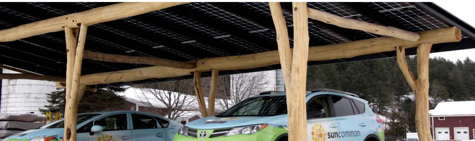
Figure 4. Black locust solar carport with a linseed based finish, approx. one month after initial application.
